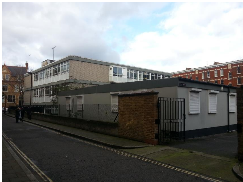
View of Shroton Street elevation (top) and view north along Stalbridge Street (bottom).
